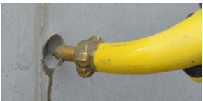
Hand pumps are an efficient and time-saving means of filling both vertical and horizontal joints and of closing fixing holes to create a void-free and rigid bond.
