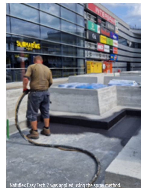
Nafuflex Easy Tech 2 was applied using the spray method.
