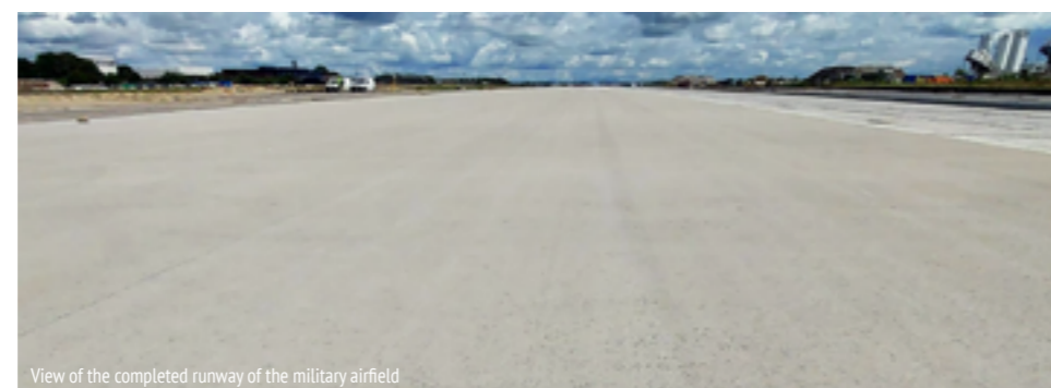
View of the completed runway of the military airfield
