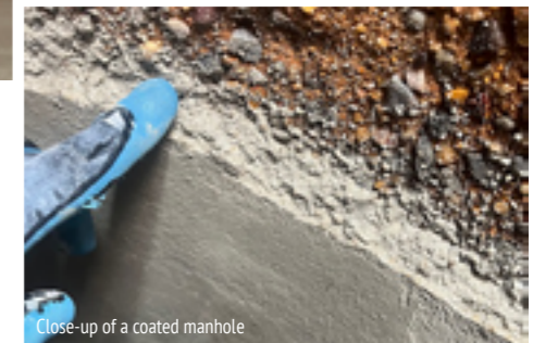
Close-up of a coated manhole
